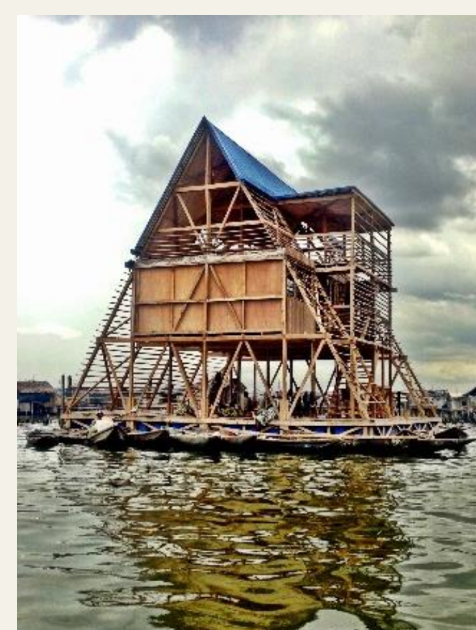
Floating School, Makoko, Lagos, Nigeria (© NLÉ)
