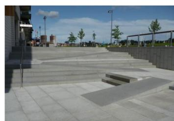
Integrated ramp into a set of stairs (Twisted Sifter, 2012)
